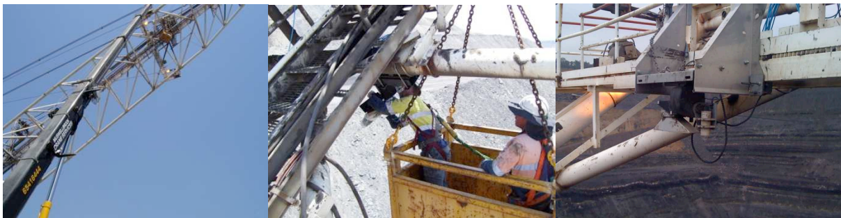
Figure 2 - Sensor Package Location, Left and centre: showing the installation to the first mounting location. Right: showing the second location on landing.
